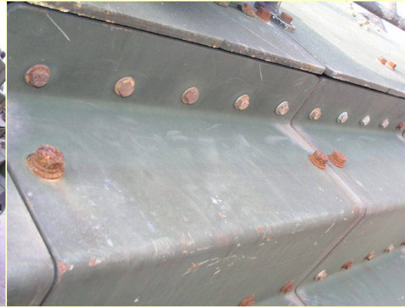
B205: Step - Thermal Spray CP-Al Inside and outside
