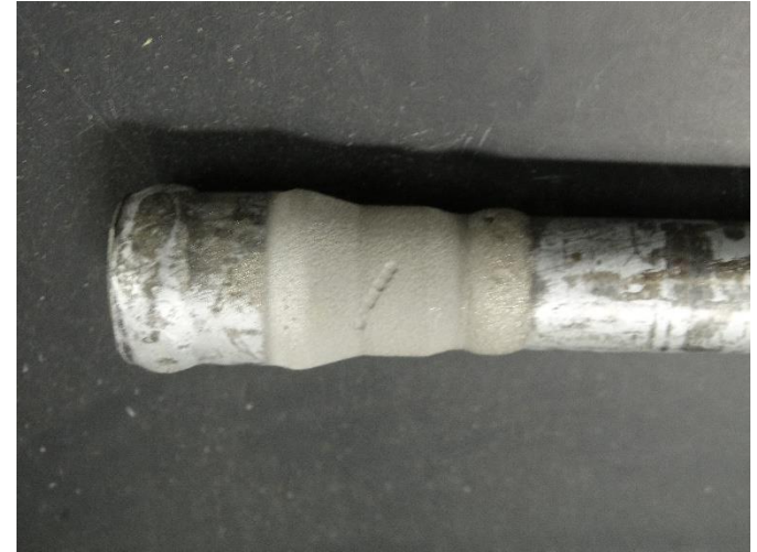
Steam Impulse Tube with Cold Spray Repair
