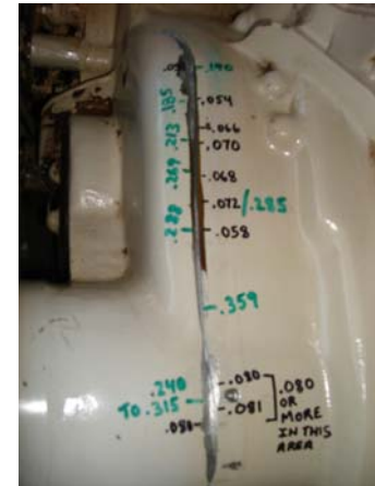
H1 C-Box Housing – Typical Damaged
